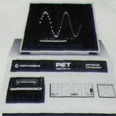
The self contained PET models 2001-4 and 8 come complete with TV screen, keyboard and built-in cassette deck as well as the computer circuitry. They are simply plugged into any 13 amp mains and no special knowledge is needed for running standard programs — over 200 of which are available on cassettes (please see separate software bulletins)
